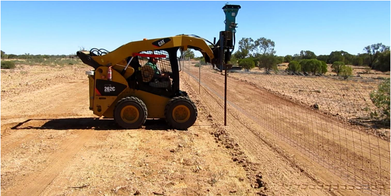
Figure 3. Drill stem being driven into the ground for in line strainers and strengtheners
