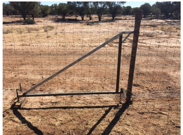
Figure 7. In line fence strainer at a 2km strain of 15/150/15 fabricated netting with temporary strut in place
