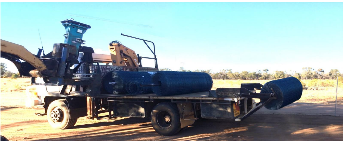
Figure 9. 15/150/15 x 500m fence rolls on truck to be rolled out on custom wire roller mounted to the back of the truck
