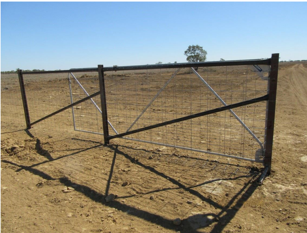
Figure 4. Strainer ends made from gauge railway line
