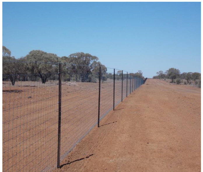
Figure 2. Completed exclusion fence with star pickets at 7m spacing and 1.6m total height
