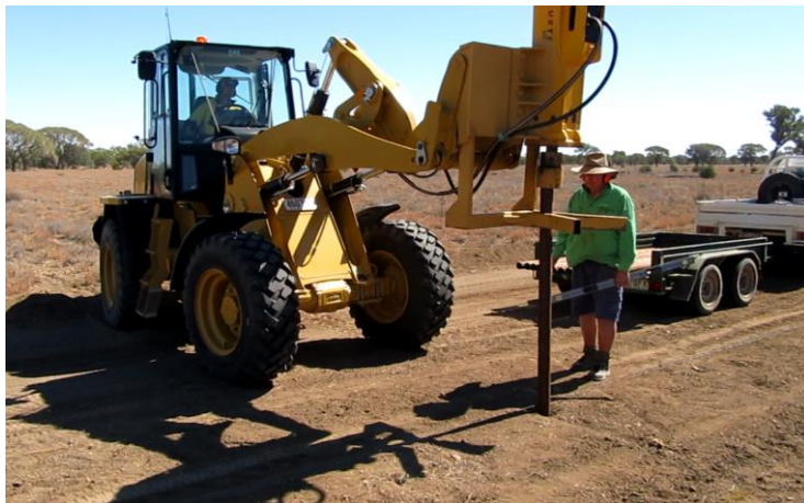
Figure 6. Front end loader with post driver/rock breaker attachment inserting an in-line strainer
